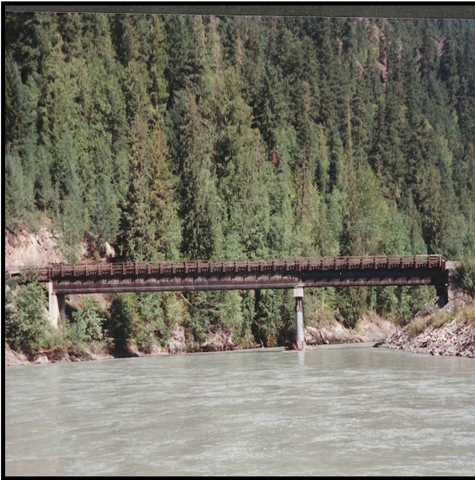
Logging bridge near Pemberton, BC
