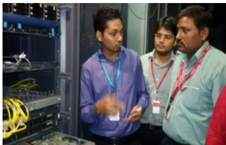
Mr. Hanuman explaining about Rack Servers
